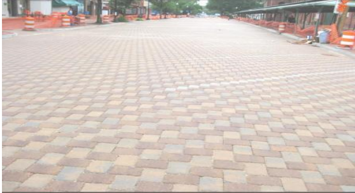
Pavers installed during the restoration of Eastern Market, 7 th Street SE
